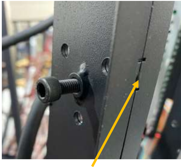
Too tight gap
